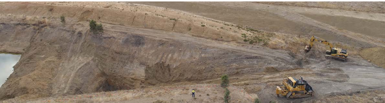
Donald Mineral Sands' Project excavation test pit.
