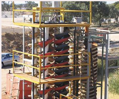
Historical wet concentrator plant pilot work, 2005.
